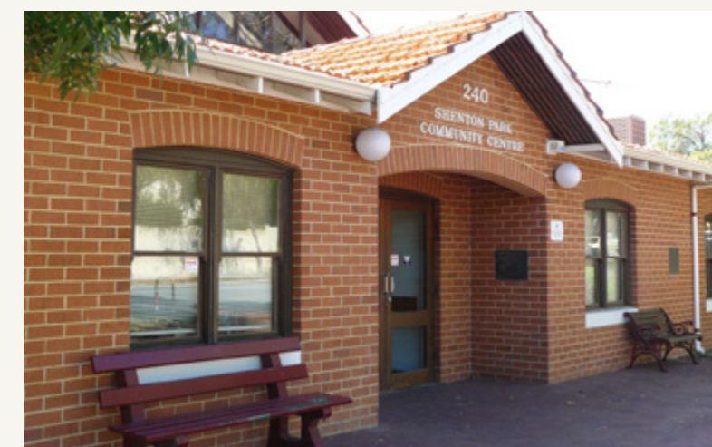
Shenton Park Community Centre
